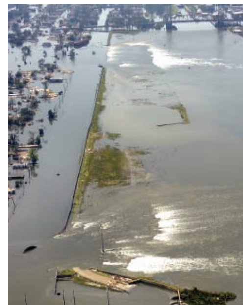
Figure 3 This levee near New Orleans broke as a result of Hurricane Katrina, allowing the Mississippi River through.
